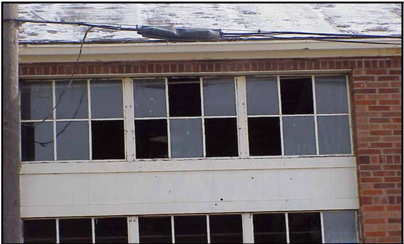
Figure 4. Vacant building south of Central Avenue West
