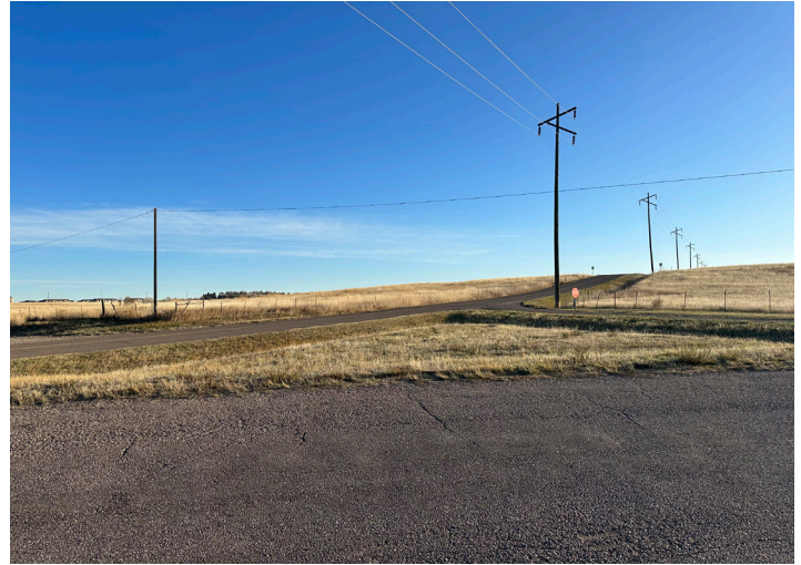
View to Northeast
