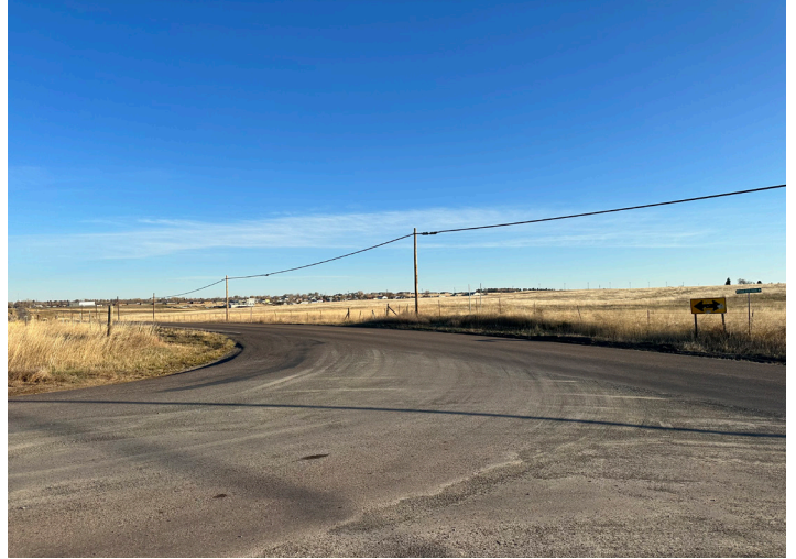
View to Northeast
