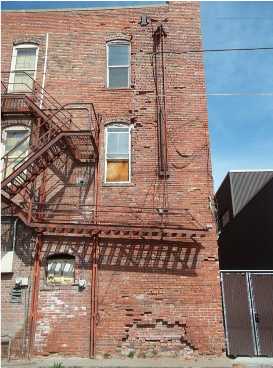
MT_CascadeCounty_BaatzBlock_0006: Alley Façade partial, showing water intrusion damage on brick veneer, looking north, July 1, 2021, photographer: Julie M. Stiteler.
