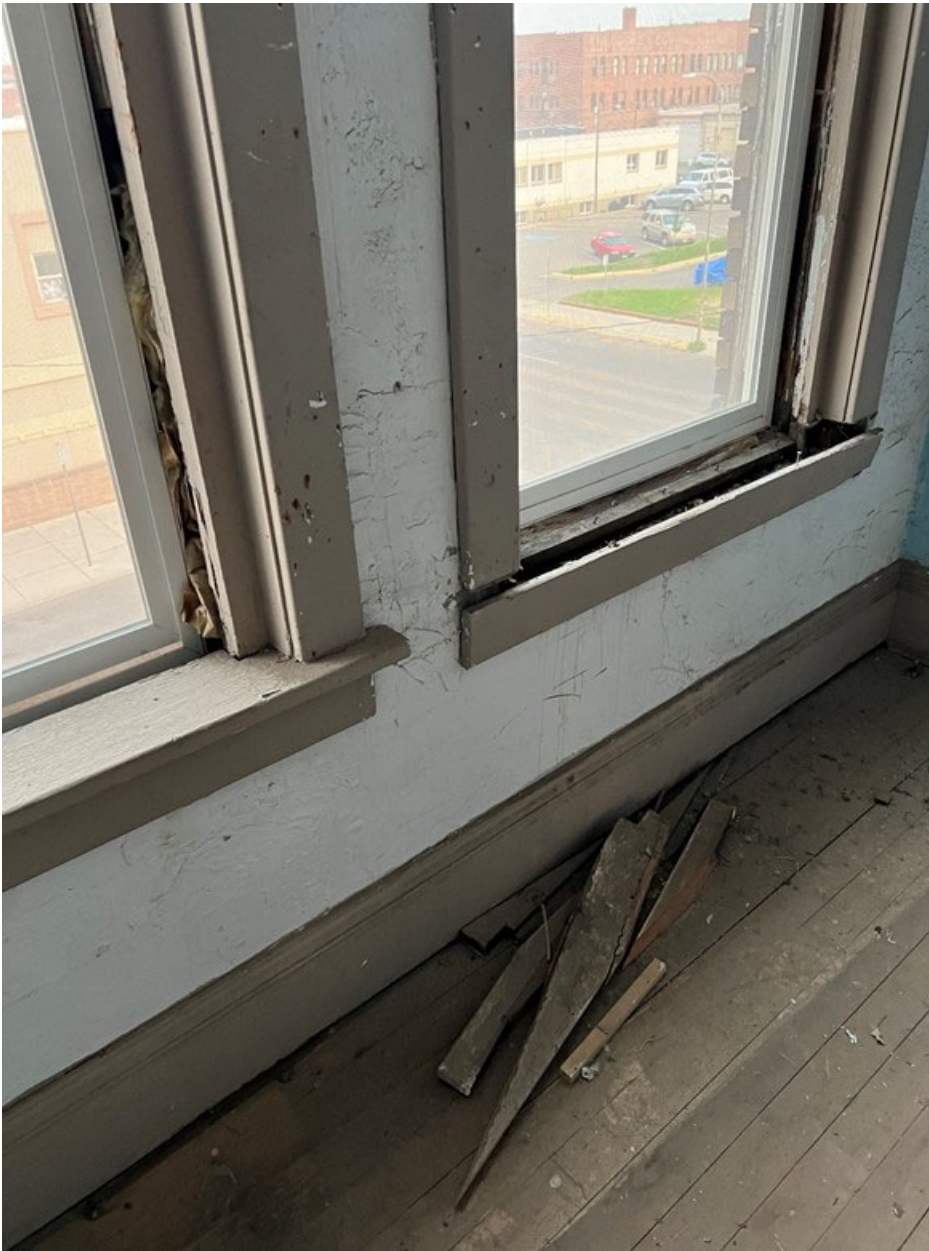
MT_CascadeCounty_BaatzBlock_0029: Replacement vinyl sash detail, showing damaged trim, looking southeast, September 11, 2022, photographer: Heather McMilin (Homeword).
