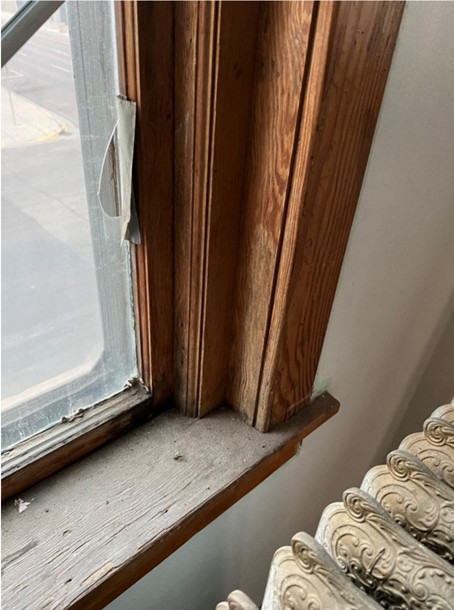
MT_CascadeCounty_BaatzBlock_0028: Original wood window detail, showing clear stain treatment on trim, looking northwest, September 11, 2022, photographer: Heather McMilin (Homeword).
