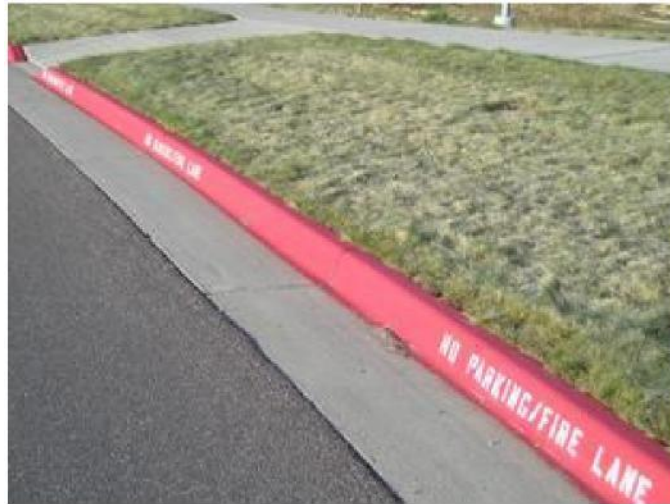
Figure 11 - Typical fire lane striping installation
