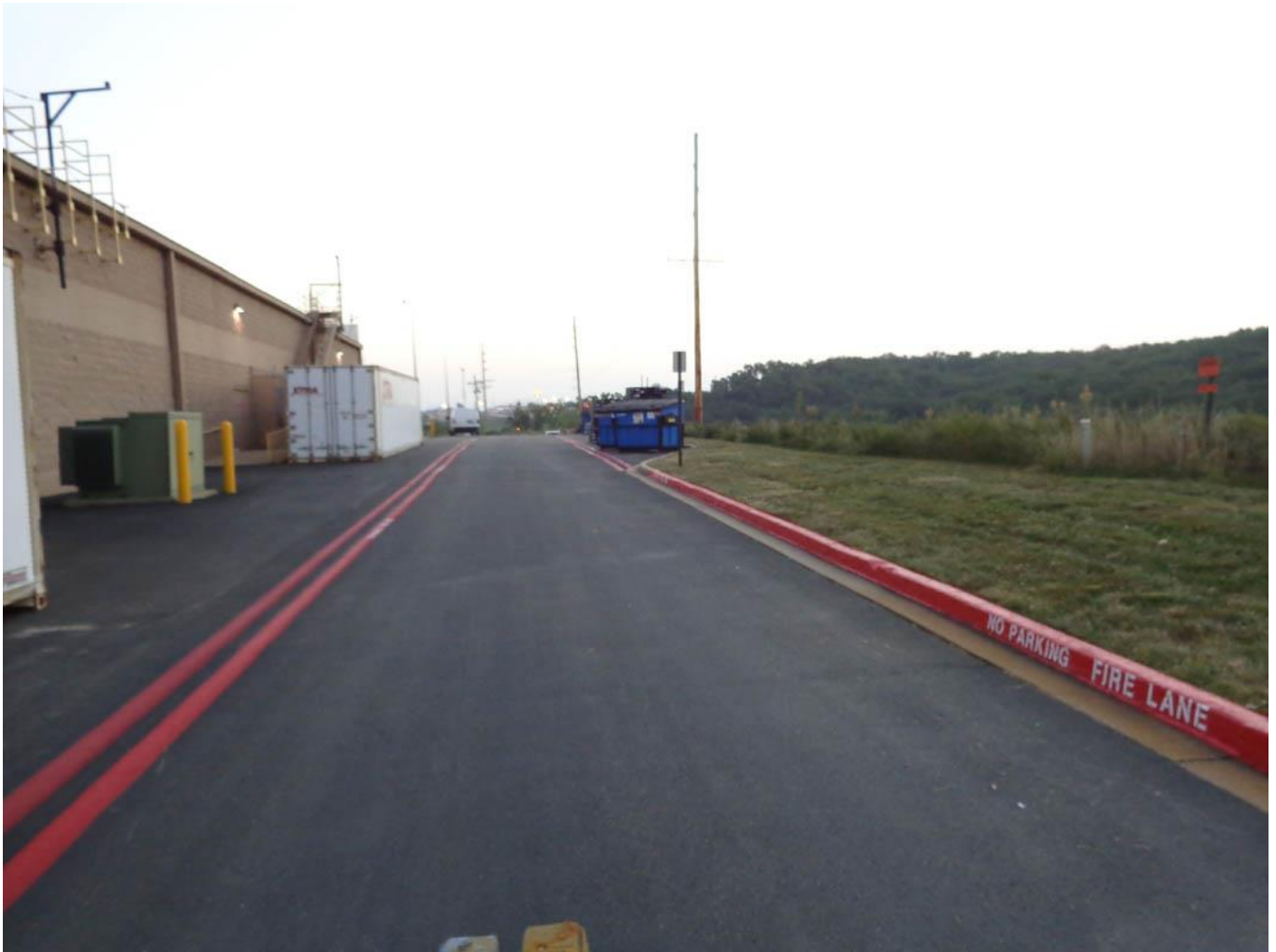
Figure 14 – Fire lane marking with pavement marking
