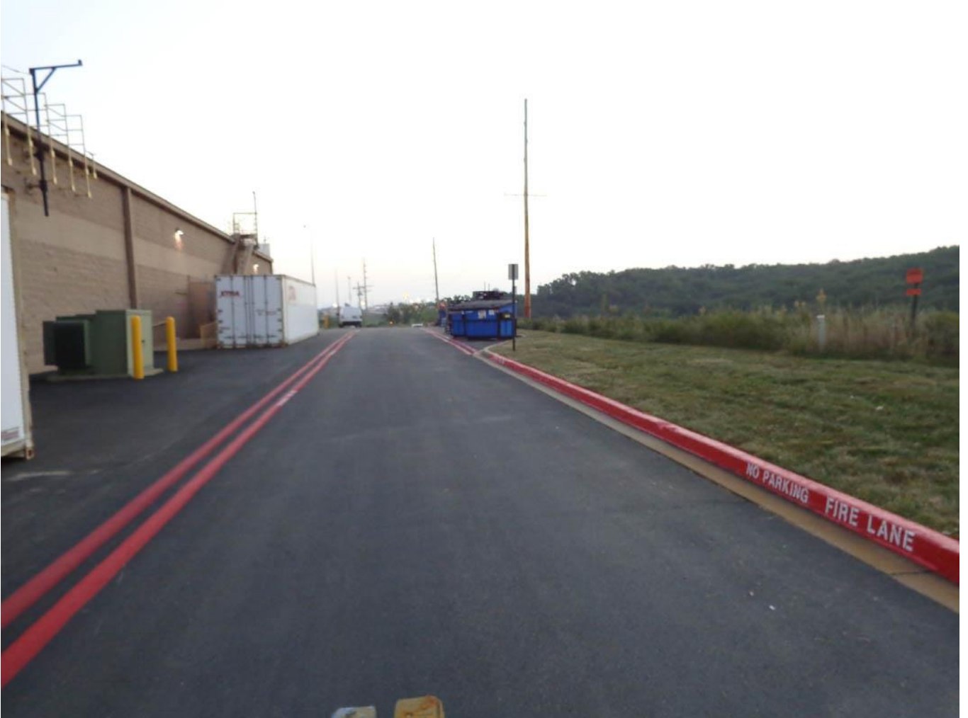
Figure 14 – Fire lane marking with pavement markings
