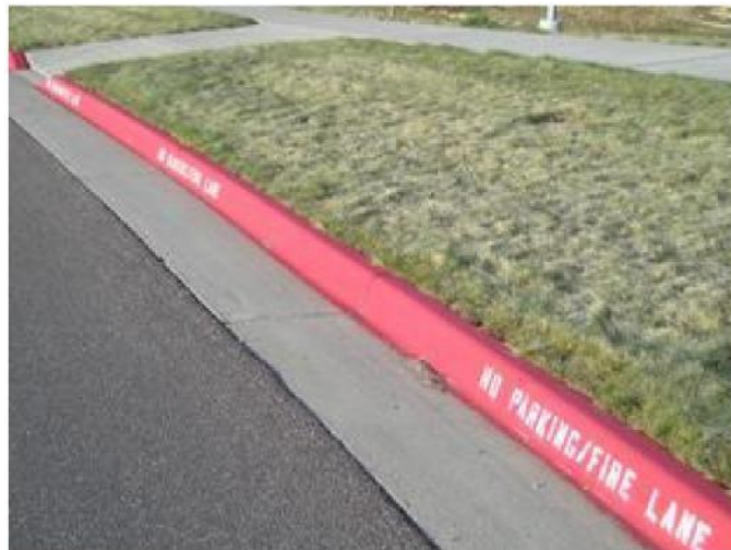
Figure 11 - Typical fire lane striping installation
