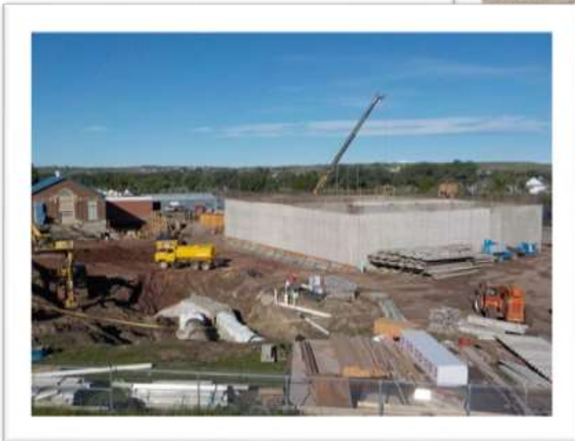
Water Treatment Plant Expansion
