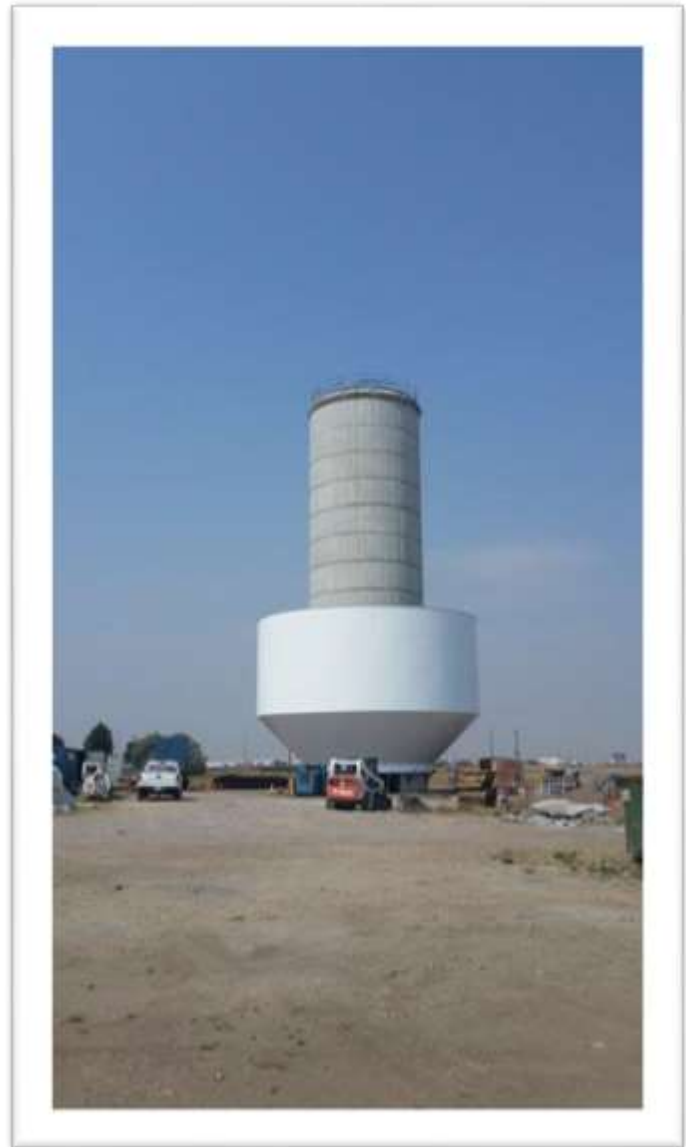
Gore Hill Water Tank Construction
