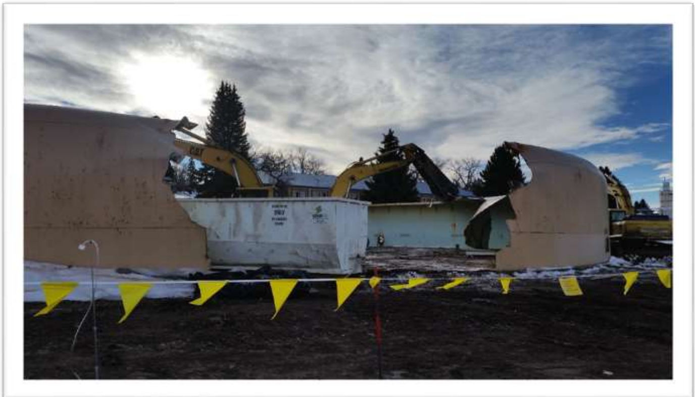
Water Tank Demolition
