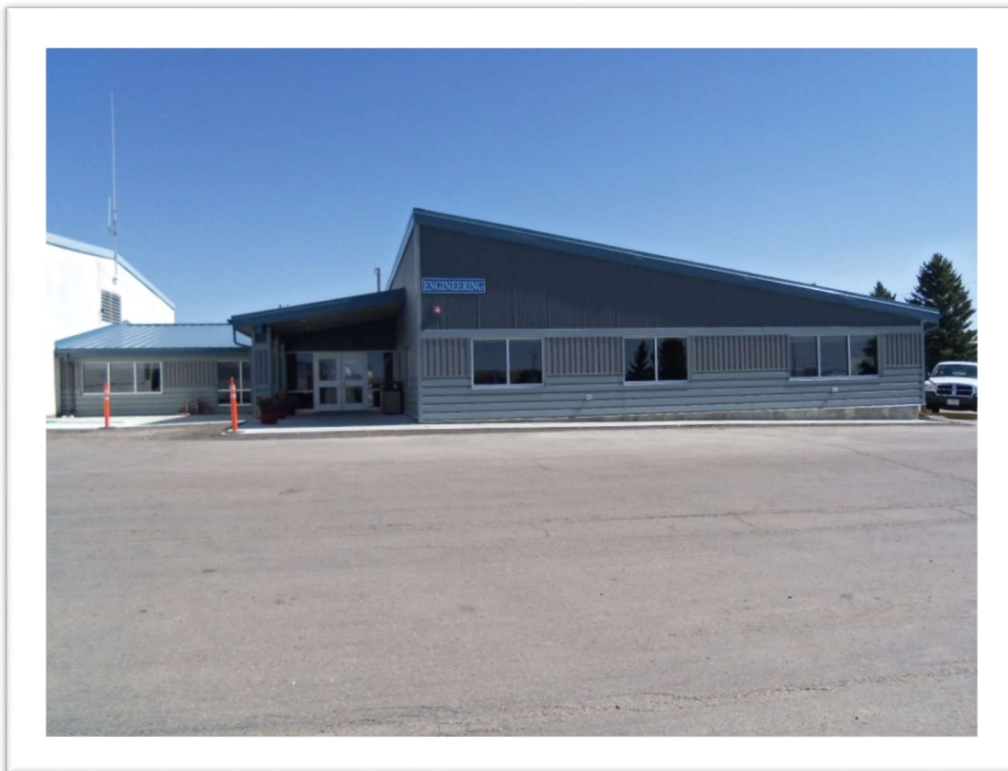
Improvements and Addition to Public Works Engineering Building
