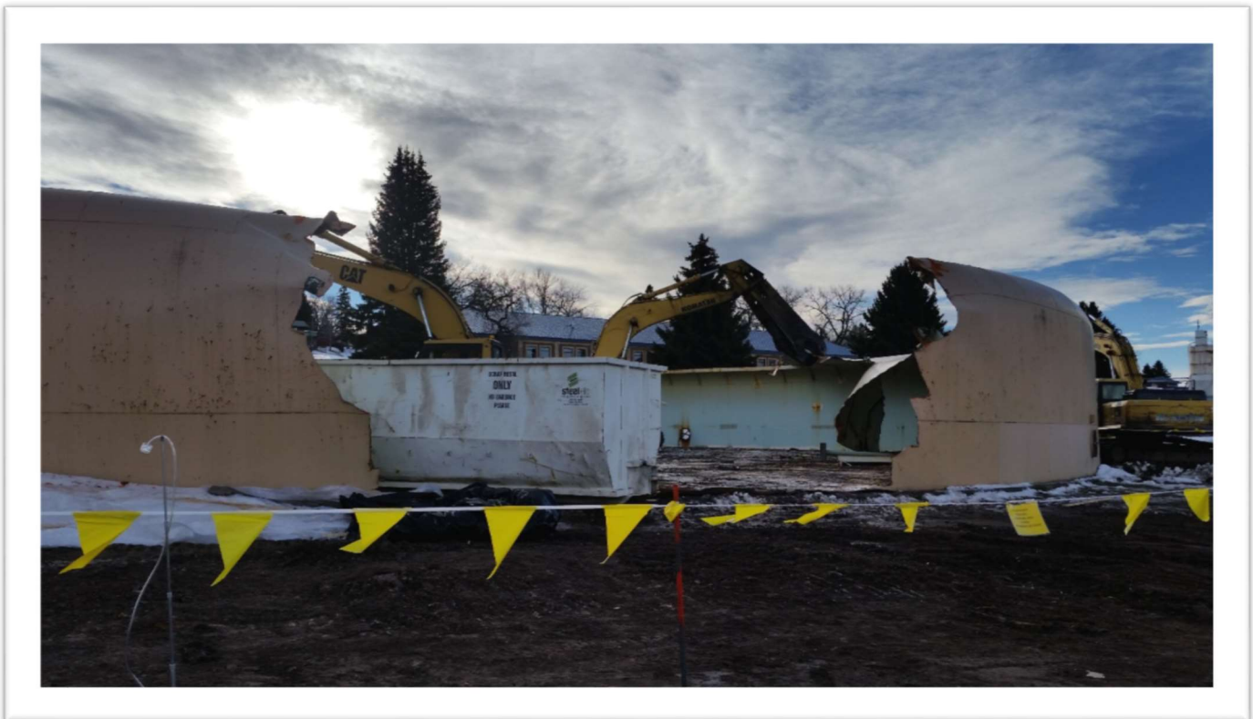
Water Tank Demolition 2018
