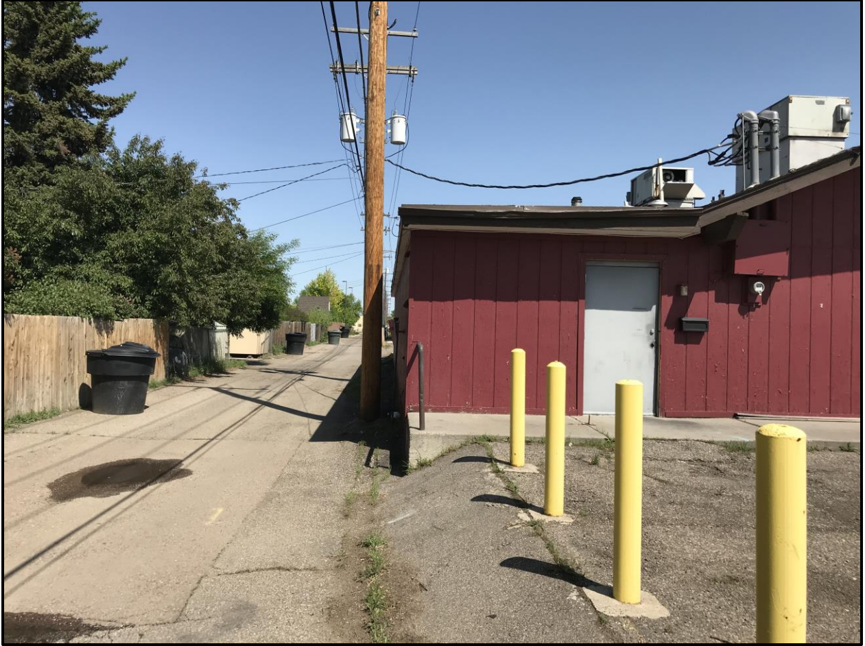
View of building relationship to alley and utilities
