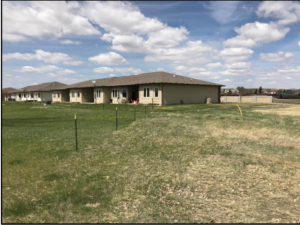
Looking West at neighboring condo complex
