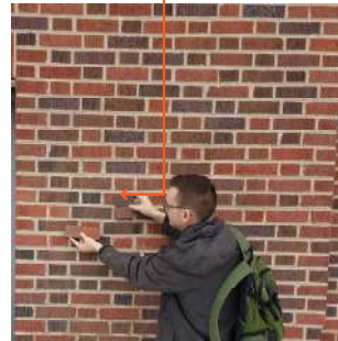
TYPICAL BRICK BLEND RUNNING BOND 70% TERRA COTTA 10% IRONSTONE 10% BRONZESTONE 10% MONTEREY RUNNING BOND, TEXTURED
