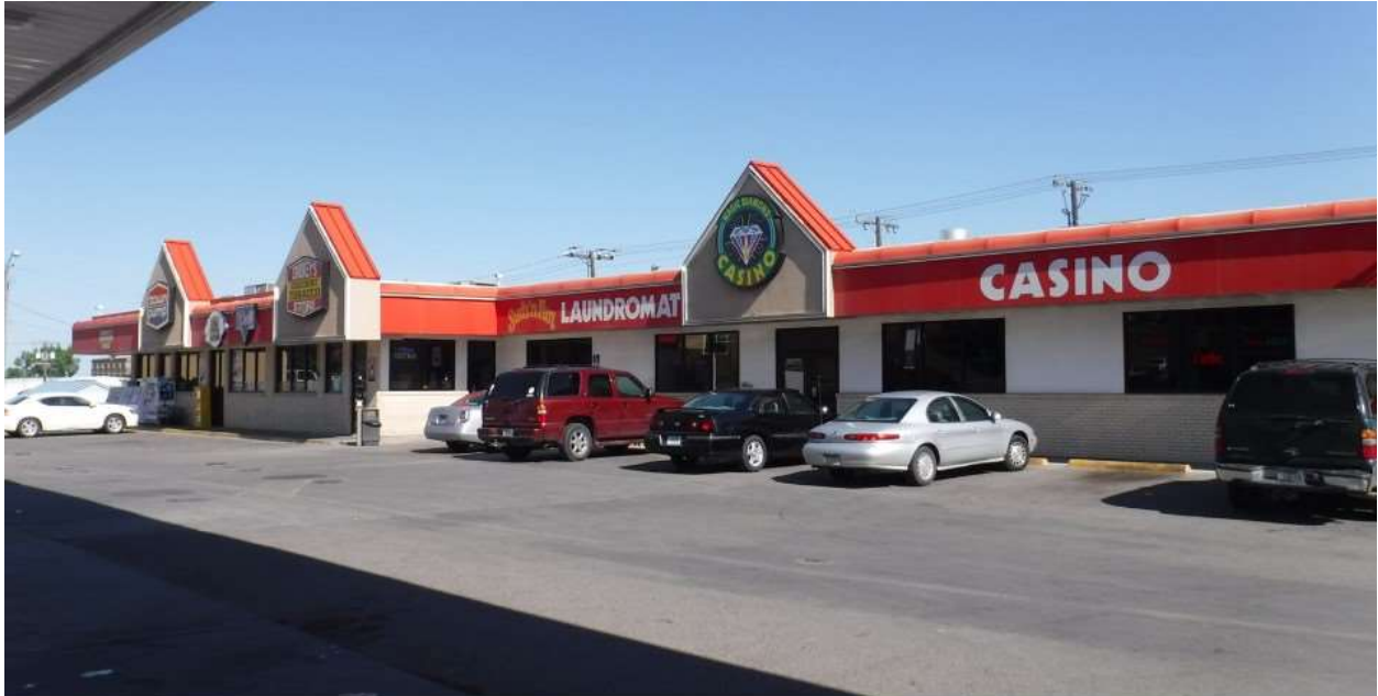
“Before” Façade of Town Pump #1 – 401 10 th Ave South
