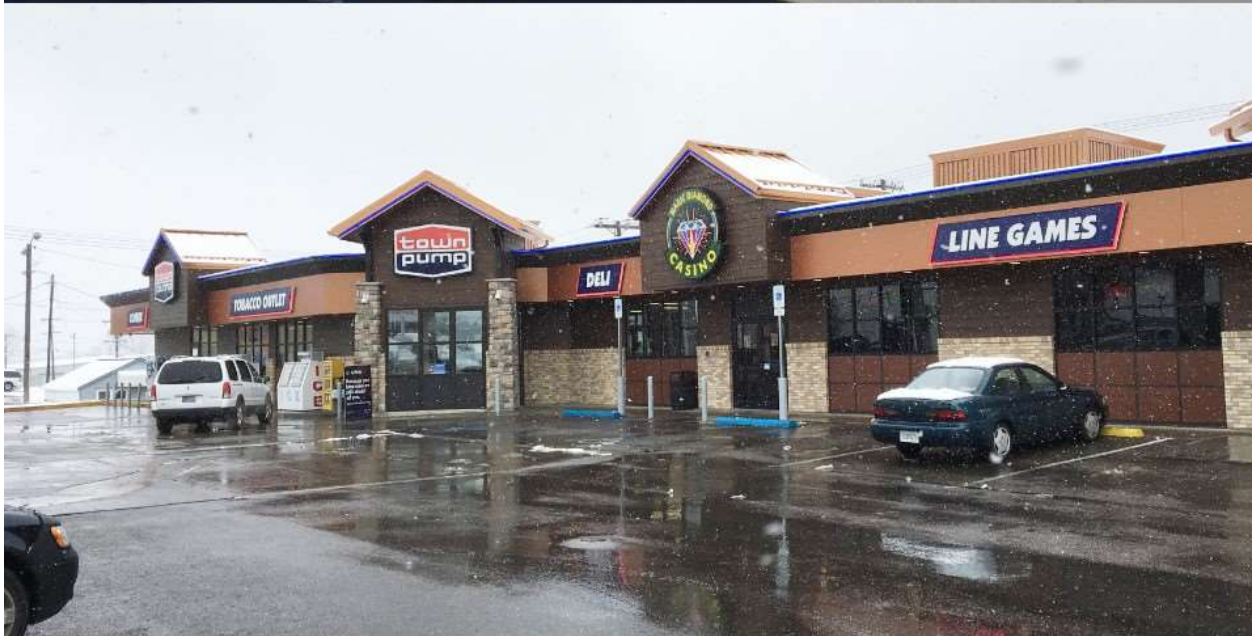
“After” Façade of Town Pump #1 – 401 10 th Ave South
