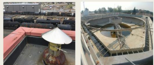
HVAC repairs on solids building ($1.1M)
