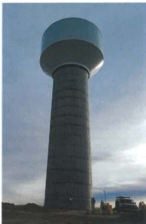
Göre Hill elevated tank near the airport. This tank has a 500,000 gallon capacity. Construction on this elevated tank was completed in 2018.
