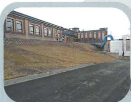
16 mixed media filters are located inside of this building.
