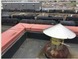
HVAC repairs on solids building ($1.1M)
