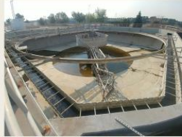
WWTP Final Clarifier Rehabilitation($4.3M)
