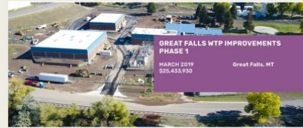
The Great Falls WTP Improvements Phase 1 project consisted of the removal of an existing above ground steel storage tank and existing piping to facilitate the construction of a new UV and Chemical Building, Surge Tank, and addition to the existing Electrical Building. Necessary site improvements included installation of new exterior underground piping from 4" to 64" diameter and a 60" and 84" bore and jack under an existing railroad spur to be the new facilities into existing.
