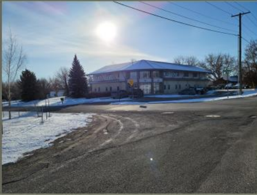
Photo – Terracon and 13 th Ave. and 14 th St. Intersection
