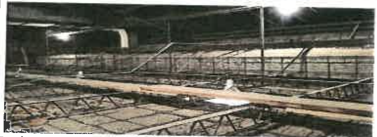
Pathways for maintaining lighting (above ceiling)
