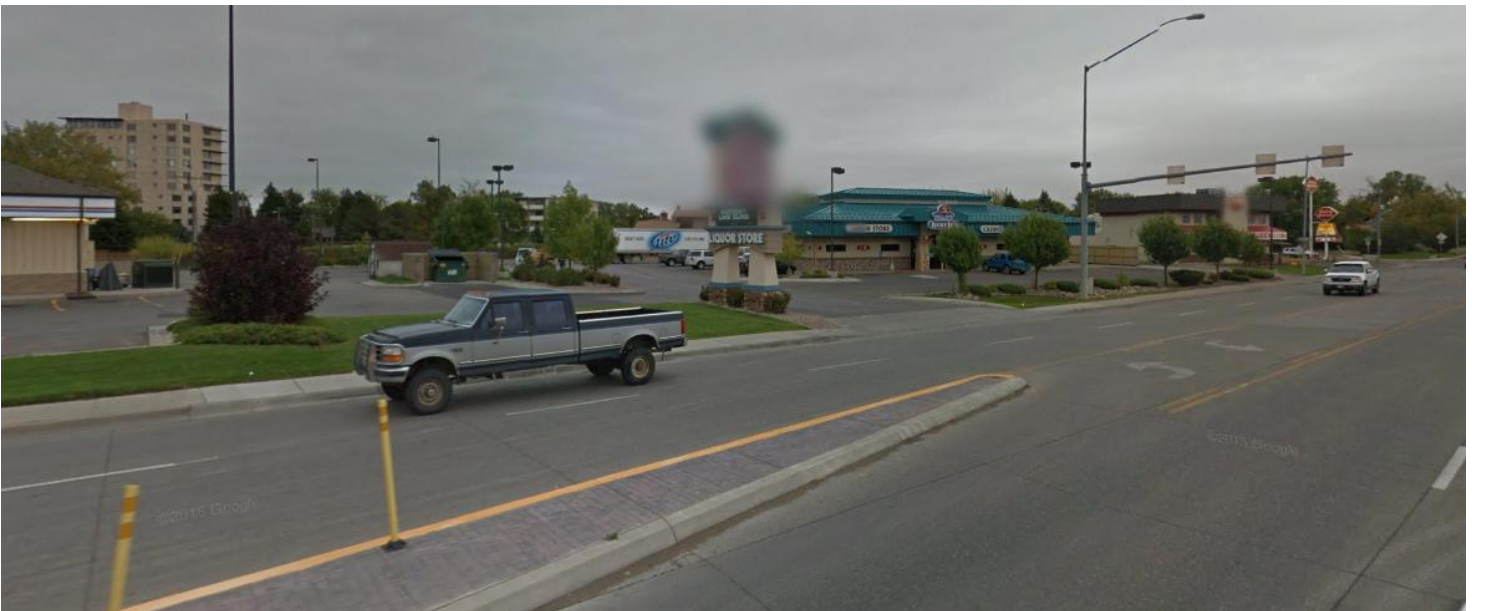
View of the existing south bound left turn pocket, which provides access to the Holiday gas station and Lucky Lil's.
