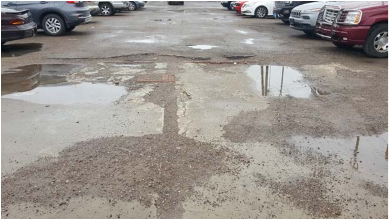
VIEW OF THE PARKING LOT SOUTH OF THE EXISTING BUILDING
