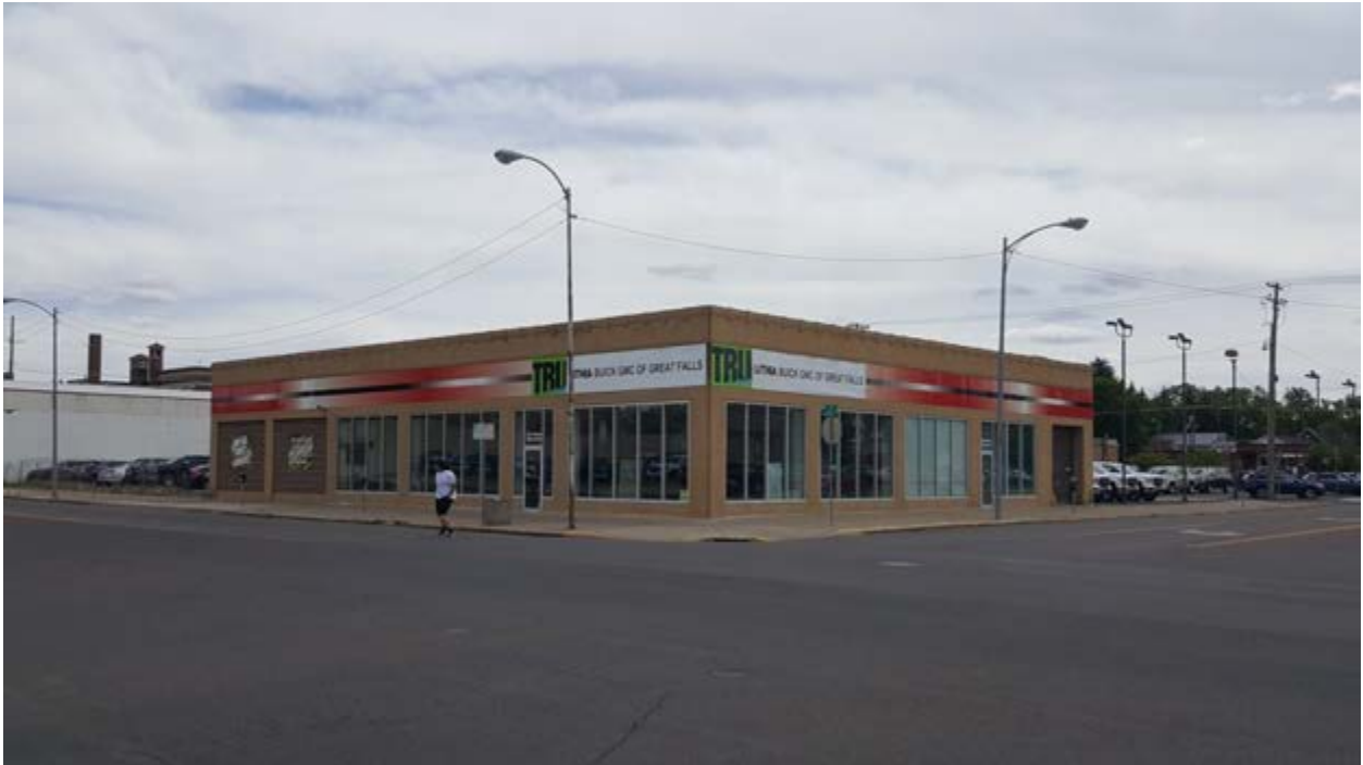
LOOKING SOUTHEAST ALONG INTERSECTION OF CENTRAL AVENUE AND 8TH STREET SOUTH
