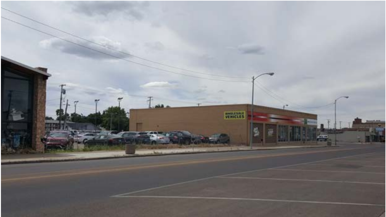
VIEW SOUTHWEST TOWARDS SHOWROOM AND CURRENT PARKING/STORAGE LOT
