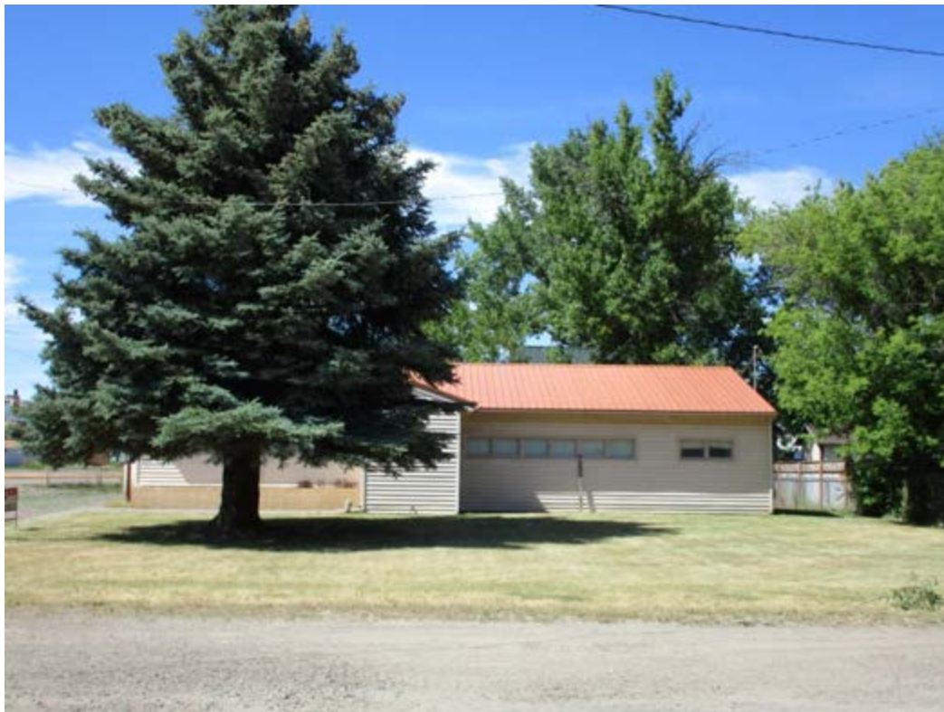
4. Looking north facing existing building; gravel on-street parking in foreground
