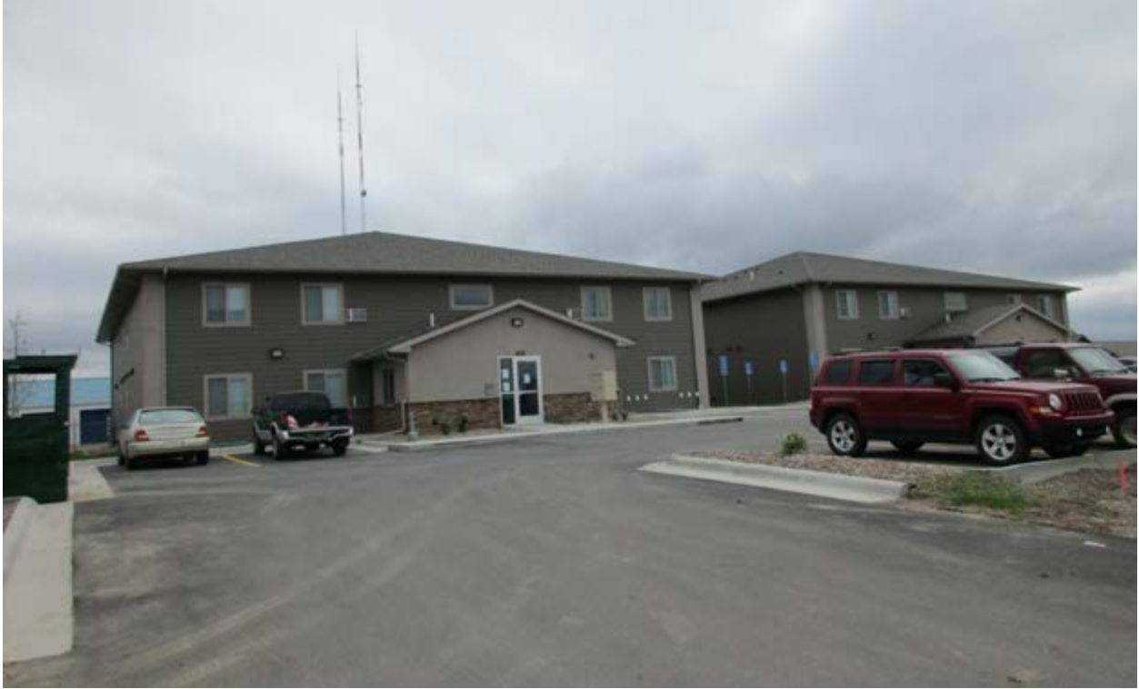
1. Looking Southwest from driveway access on 36th Avenue Northeast.
