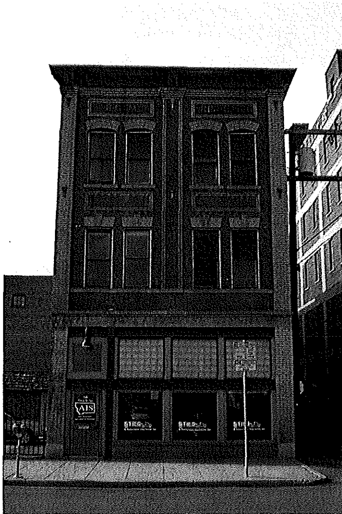
EAST EXTERIOR FAÇADE
