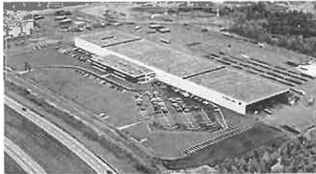
Head office and new fabrication plant in Terrebonne (1997)
