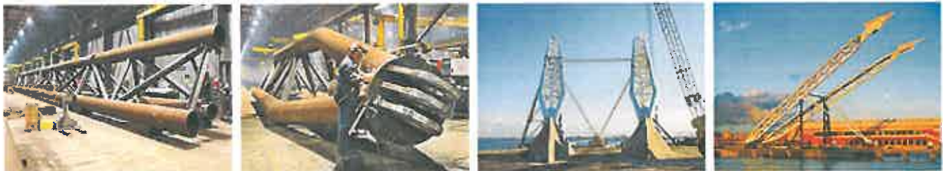
Pier Steel Structure (Port of San Juan, Puerto Rico)
