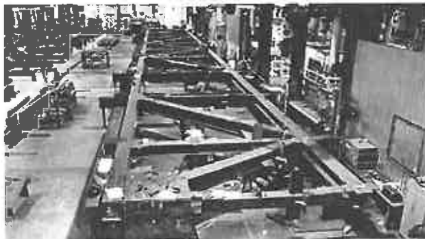
Trial-assembly of an oversized steel truss of the tower (New York, NY, U.S.A.)
