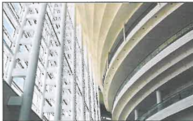
Miscellaneous and architectural metals Balconies and steel/glass atrium of the Carnival Performing Arts Center, in Miami
