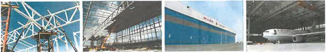
Boeing 747 Maintenance Hangar for Air Algeria (Algiers, Algeria, North Africa)
