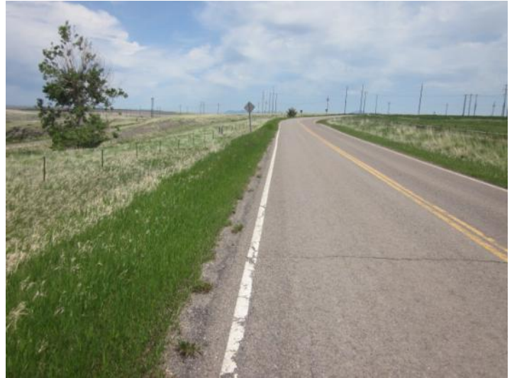
View east along Giant Springs Road with subject property on right
