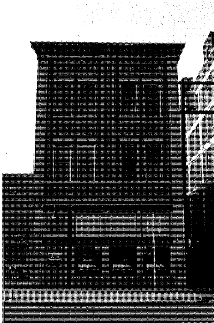
EAST EXTERIOR FAÇADE
