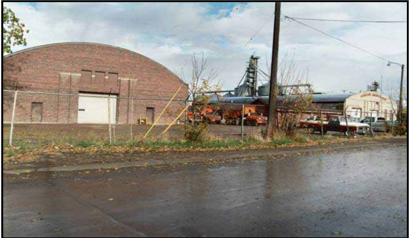
Figure 2 Cascade County Shops
