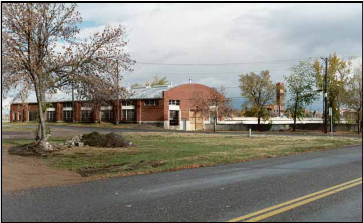
Figure 4. Former Highway Department Building
