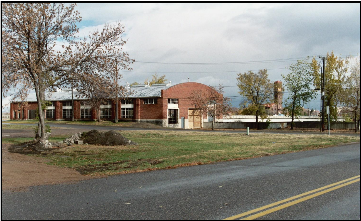
Figure 4. Former Highway Department Building
