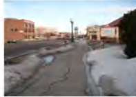
Poor Street & Sidewalk Maintenance
