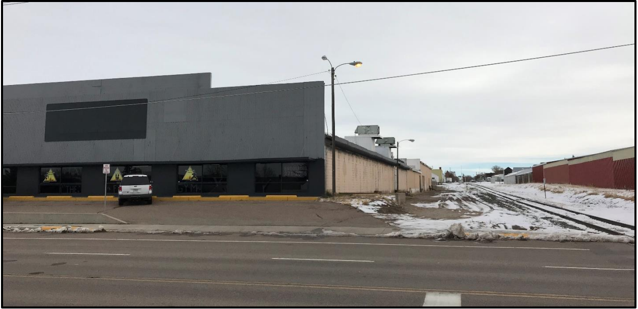
Looking east at southern portion of building and BNSF Right-of-Way
