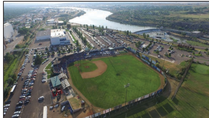
It is recommended that Great Falls review access to the Voyagers ballpark and develop a plan to manage traffic into and out of the ballpark.
