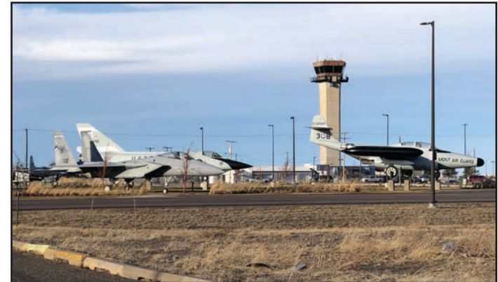
The Great Falls International Airport has substantial infrastructure for the air cargo industry.
