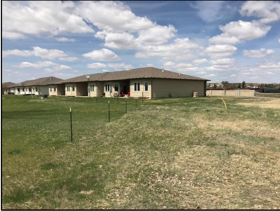
Looking West at neighboring condo complex
