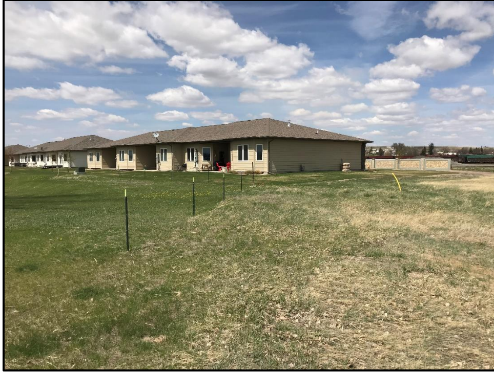
Looking West at neighboring condo complex
