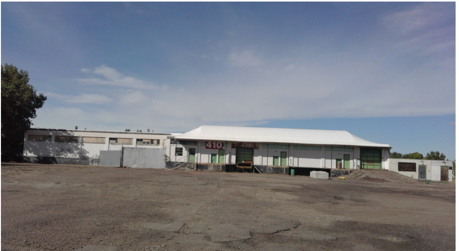
Looking west from 14th St SW towards existing warehouse.
