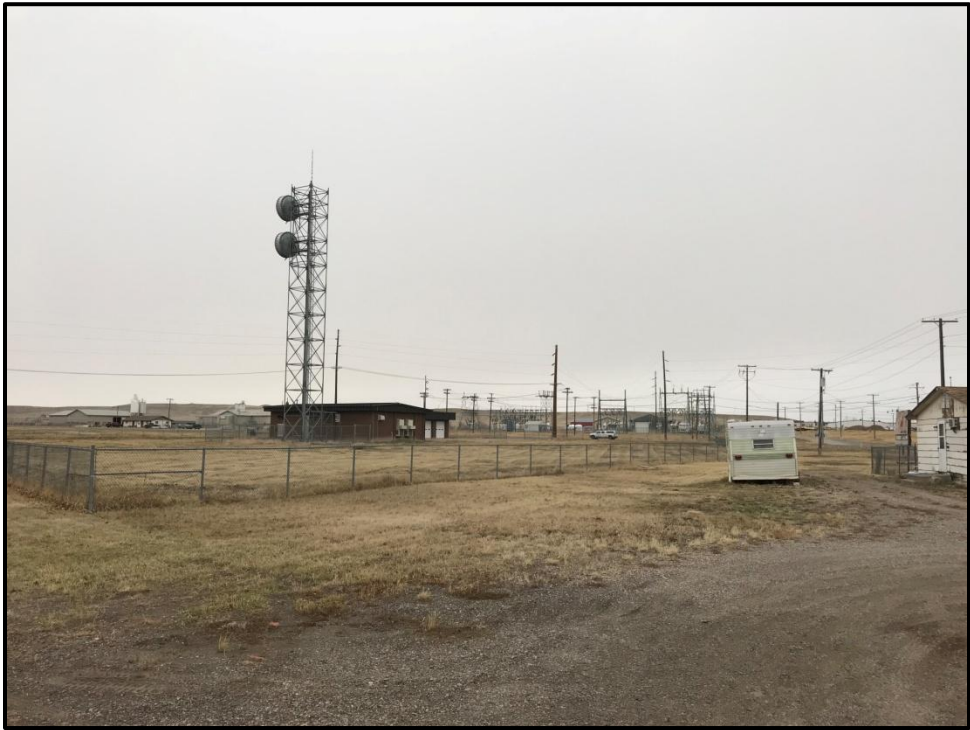
View looking Northwest from alley
