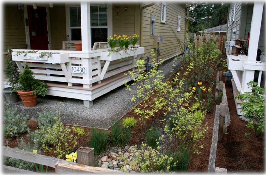
Storm water from roofs is directed into rain gardens - small vegetated swales alongside most homes - part of a “low-impact development” program. Storm water filters back into the ground through drainage swales in the pocket neighborhood greens.
