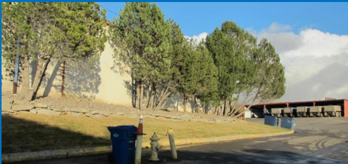
Public Works Complex Irrigation Improvements; Storm Water BMP
