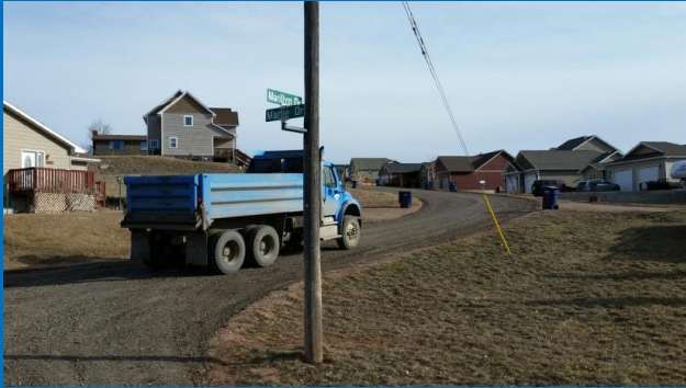
Recycled Asphalt Screenings were used to improve road surfaces in the Pearson Addition.
