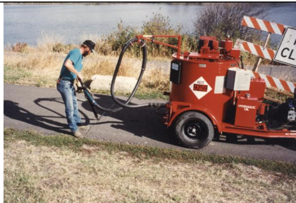
Typical Maintenance Activity - Annual crack sealing of asphalt trails
