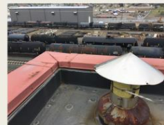
HVAC repairs on solids building ($1.1M)
