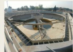
WWTP Final Clarifier Rehabilitation ($4.3M)
