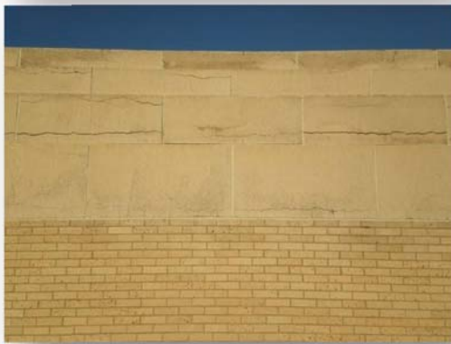
Various Degrees of Cast Stone Deterioration
