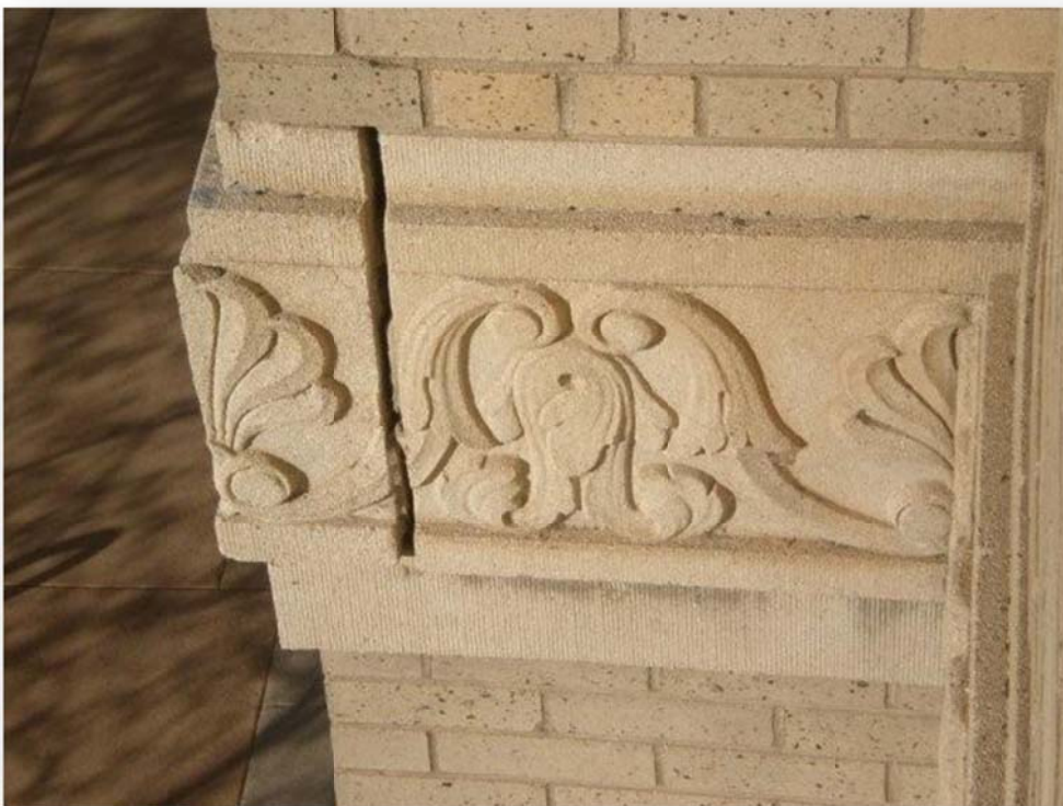
Photo S8 – Typical Weathered Mortar Joint
