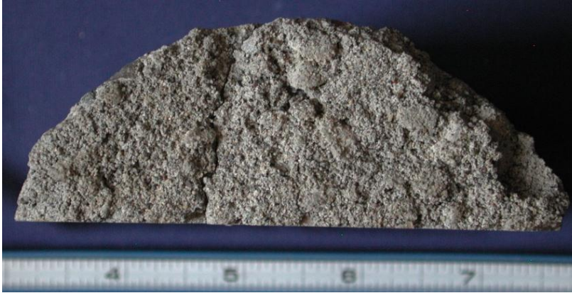
Figure 7. View of the inner, poorly densified surface of the backup concrete.
