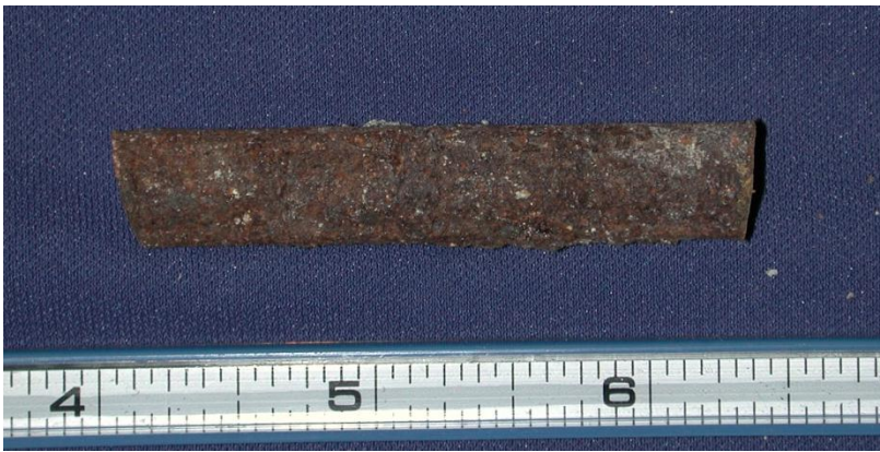
Figure 8. Section of the corroded reinforcing bar.
