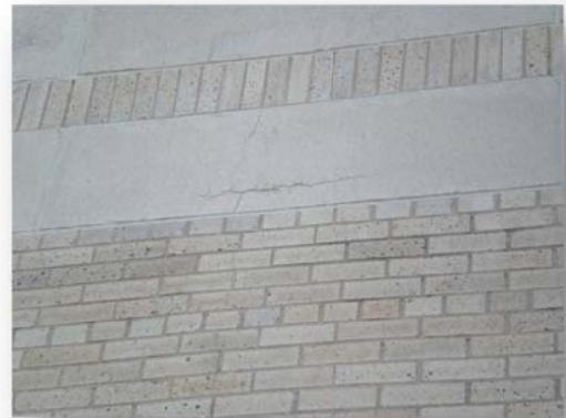
Fine Cracking
