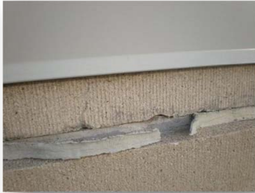
Caulking Over the Top of Mortar Joint
