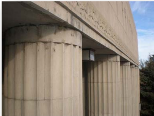
Fluted Columns on East Façade
