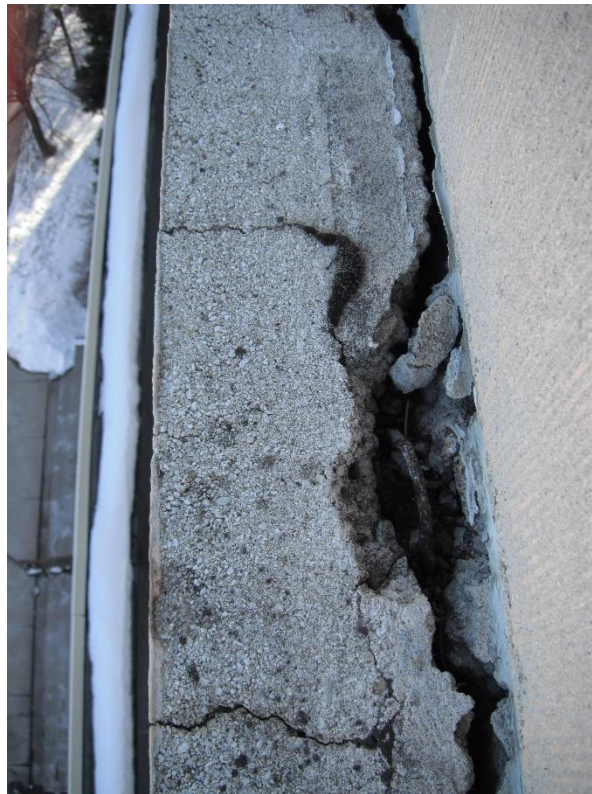
Figure 8 - Exposed Reinforcement
