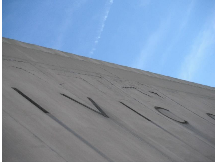
Figure 3 - Some Panels Exhibit Potential for Shearing due to Internal Forces
