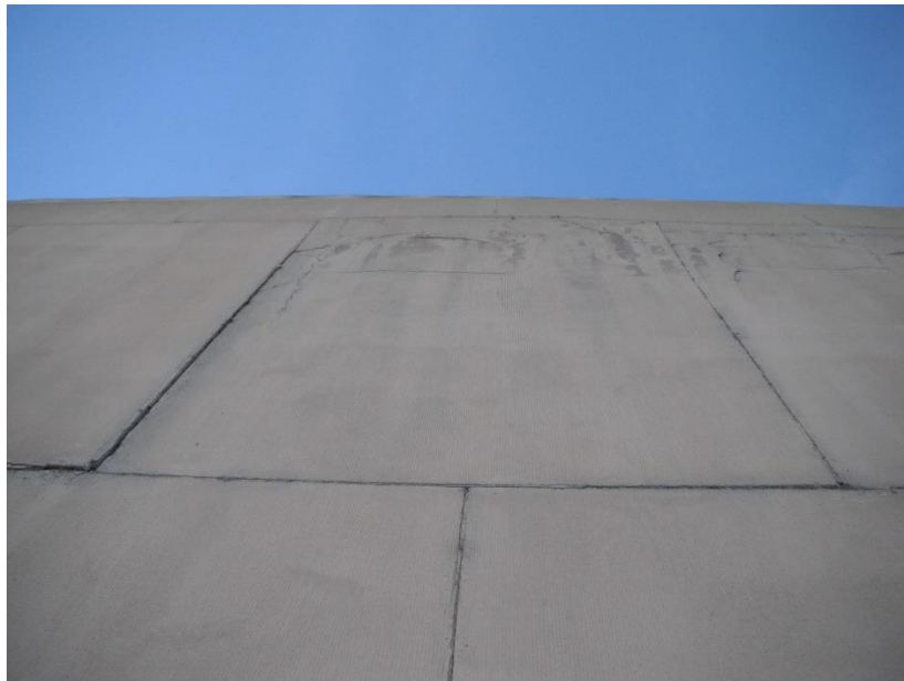
Figure 2- Surface Cracking
