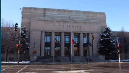
Civic Center Façade Project
