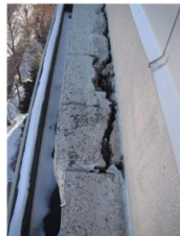
heavy separation and entry points for air and water
