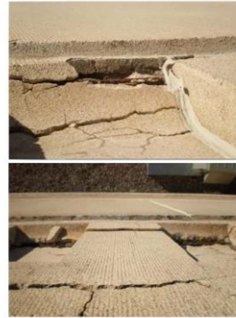
deterioration of the exterior and lack of mechanical attachment
