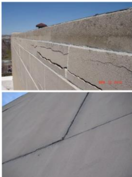
heavy separation and entry points for air and water
