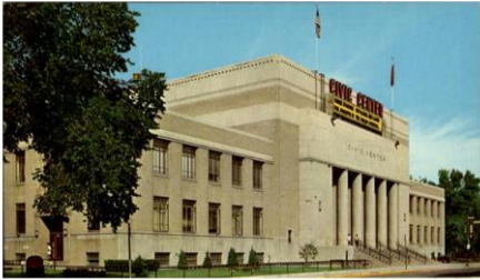
Great Falls Civic Center Exterior Envelope - A Review
