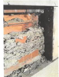
deterioration of the exterior and lack of mechanical attachment
