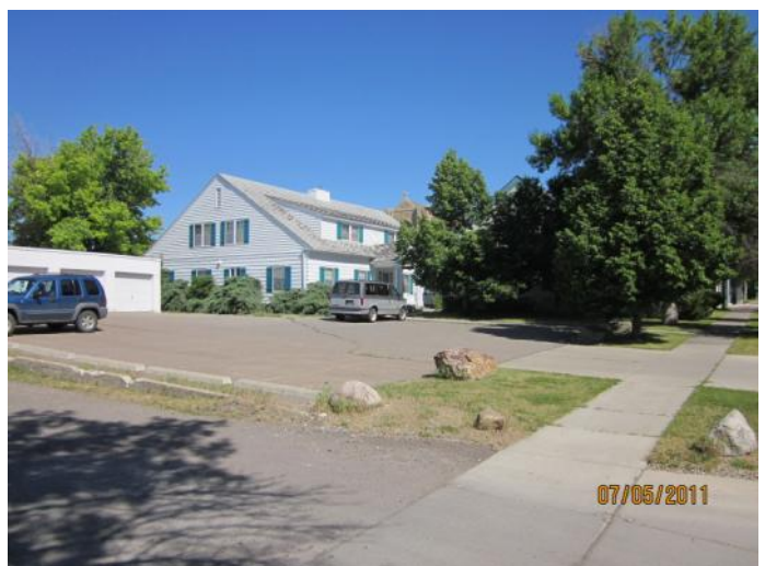
View looking north from 1st Alley South at the four-unit multi-family structure.
