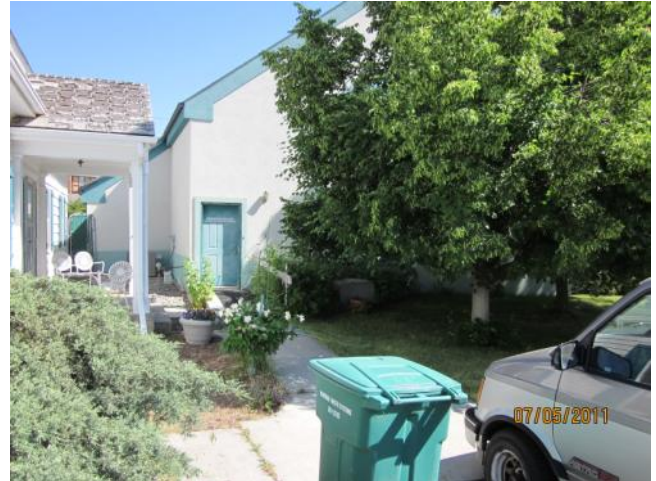
View looking at the existing rear entry of the commercial structure.
