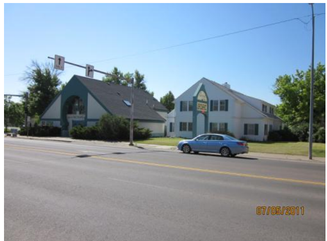
View looking west at the front of the existing structure.
