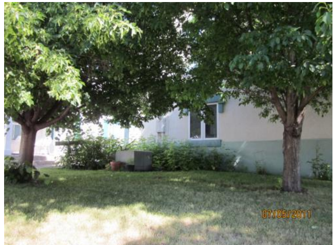
View looking at the south elevation of the commercial structure and the two trees to be removed.
